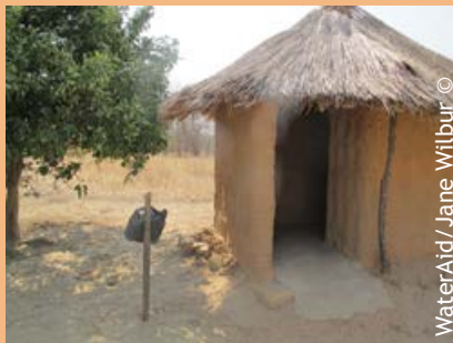
Marina's inclusively designed toilet with a handwashing facility outside the toilet
